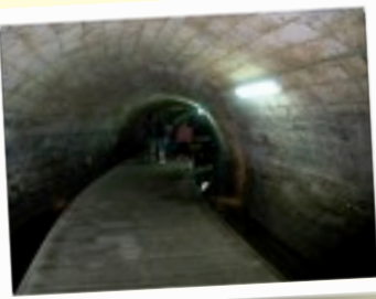
Templer Tunnel water system
